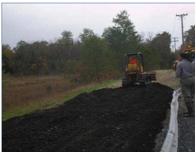
Roadside spreading of compost by NYSDOT.
